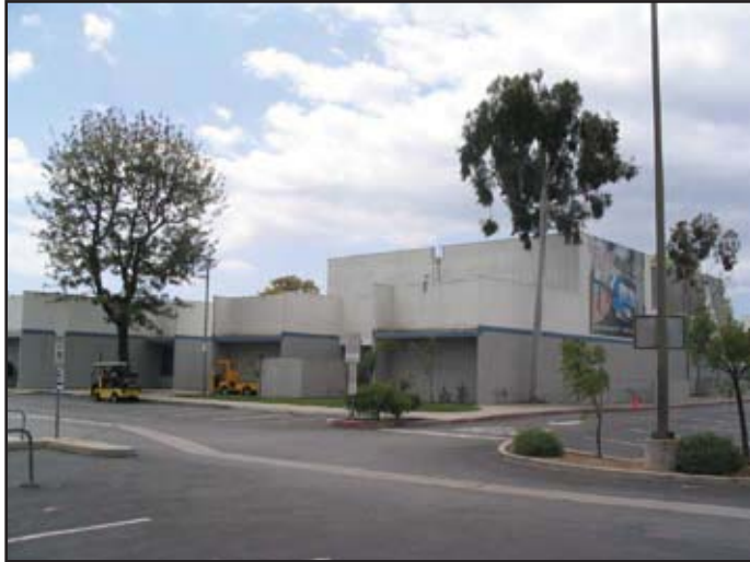
View 18: View from the northeast corner of the Project Site looking southwest at the Concert Hall.
