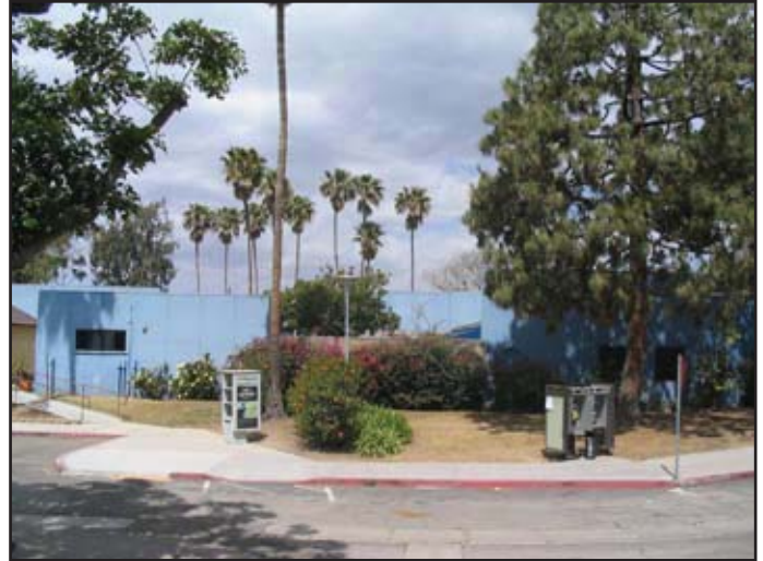
View 10: View from the Project Site looking north at the south side of the Admissions/Student Services Complex.
