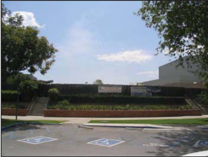
View 12: View from the Project Site looking south at the north side of the Amphitheater.
