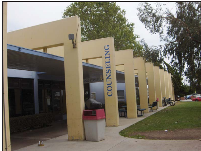
View 3: View of the Counseling Complex. The boxy one-story building is horizontally oriented with a flat roof. The windows are arranged in panels, forming a grid.
