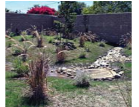
Bioswale at Bundy Campus
