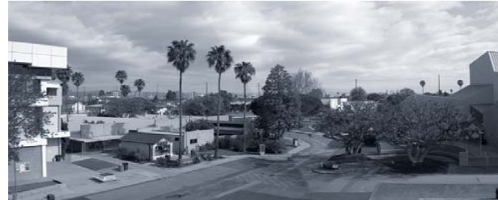
View from HSS building looking at proposed Student Services Building location.
