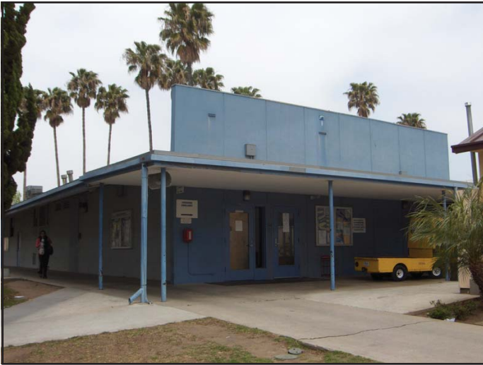
View 1: View of the Admissions and Student Services Complex. Each building is a plain rectangular box covered by a flat roof with overhanging eaves.
