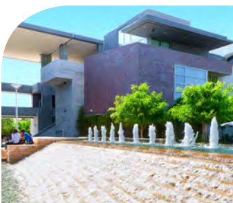
HSS Building / Quad
