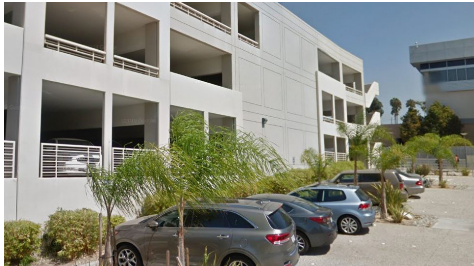
Vehicle Parking in Parking Structure Four
