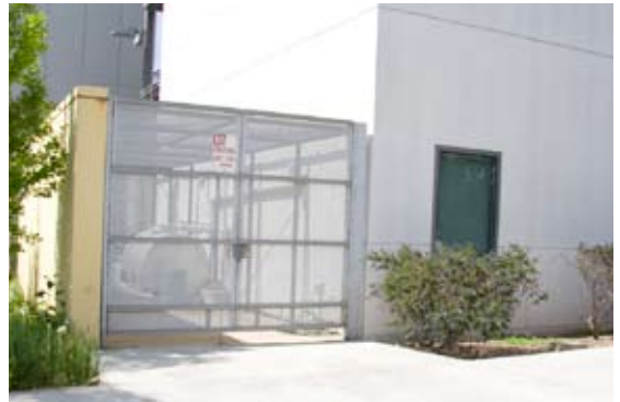
Utility zone at the Science Complex.
