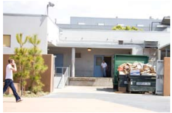
Service zone at the Bookstore/Health Service/Cayton Center & Cafeteria.
