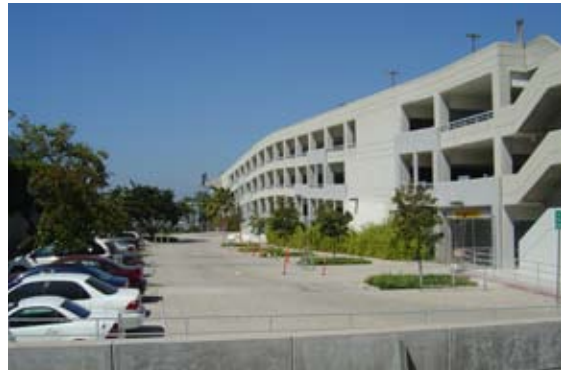
Fire lane north of the Business Building.
