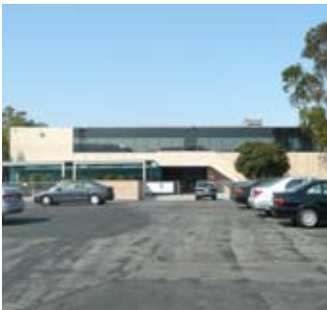
Primary access from parking lot to the AET Building.
