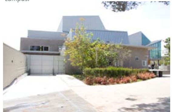
Service and utility access at Theater Arts.
