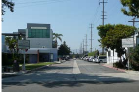
Fire lane east of the Life and Physical Science Complex.
