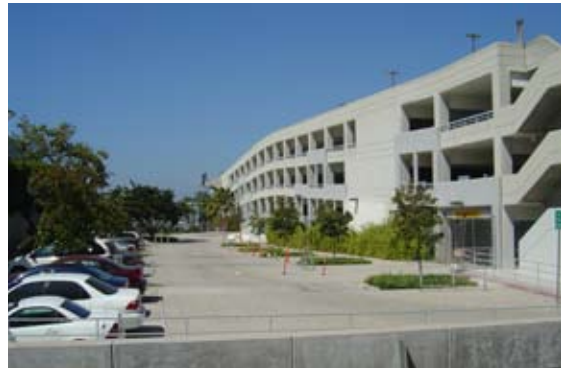
Fire lane north of the Business Building.
