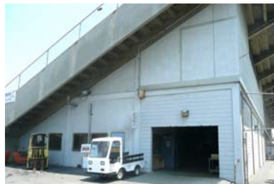
Access to the service and utility zone at Corsair Stadium.
