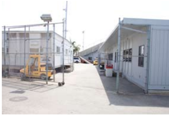
Service and utility zone at Corsair Stadium.
