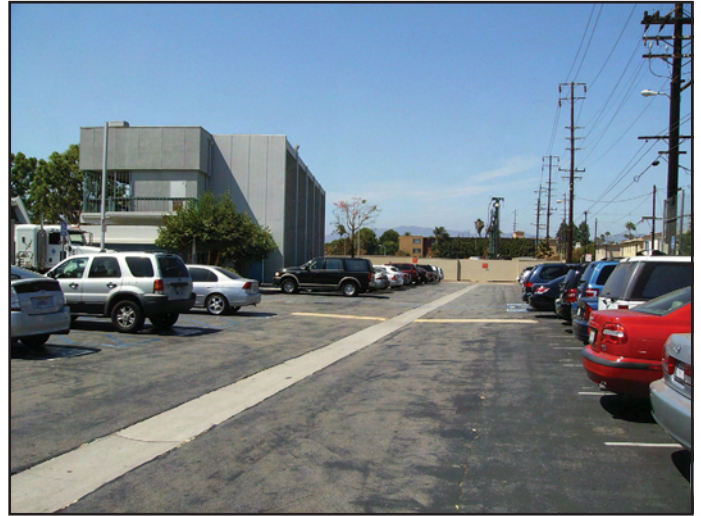
View 20: View looking northwest along the east parking drive toward the Art Complex and construction wall.
