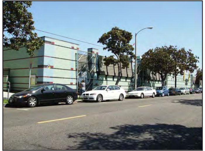
View 6: Looking southeast across 16th Street toward the Santa Monica Swim Center located along the Main Campus frontage.
