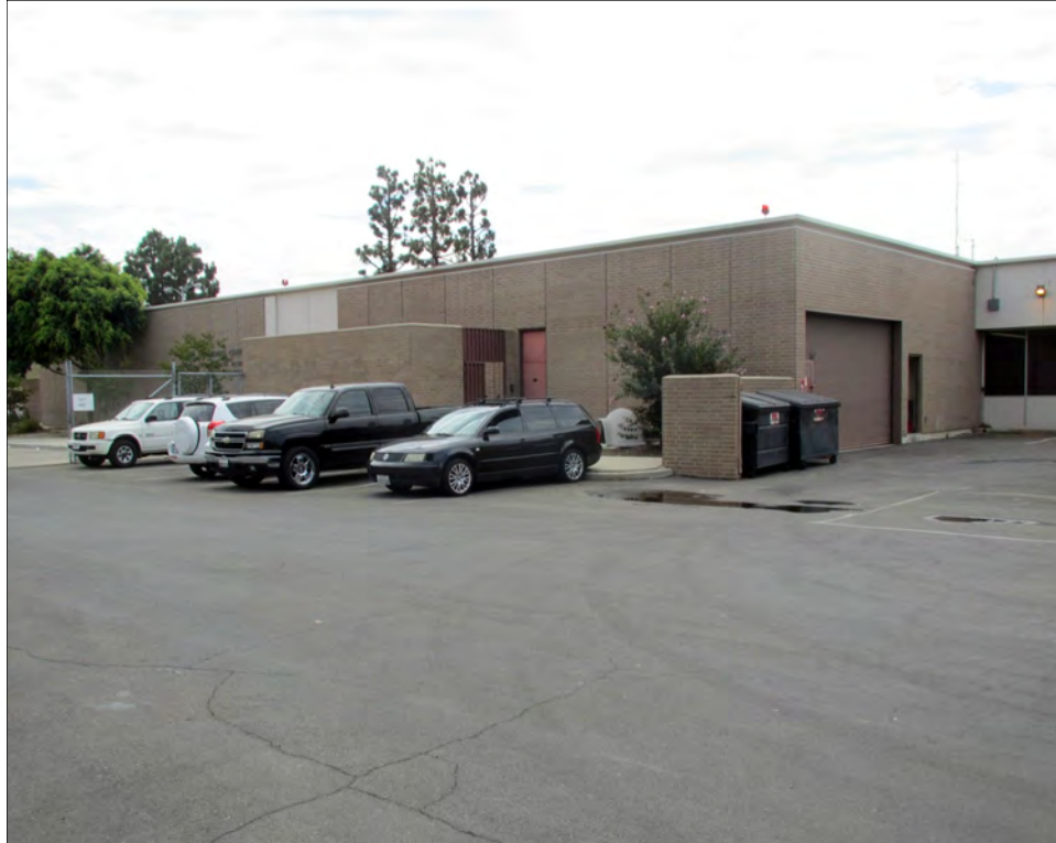
Figure 28: Courthouse, north elevation, view southeast (Heumann, 2015)
