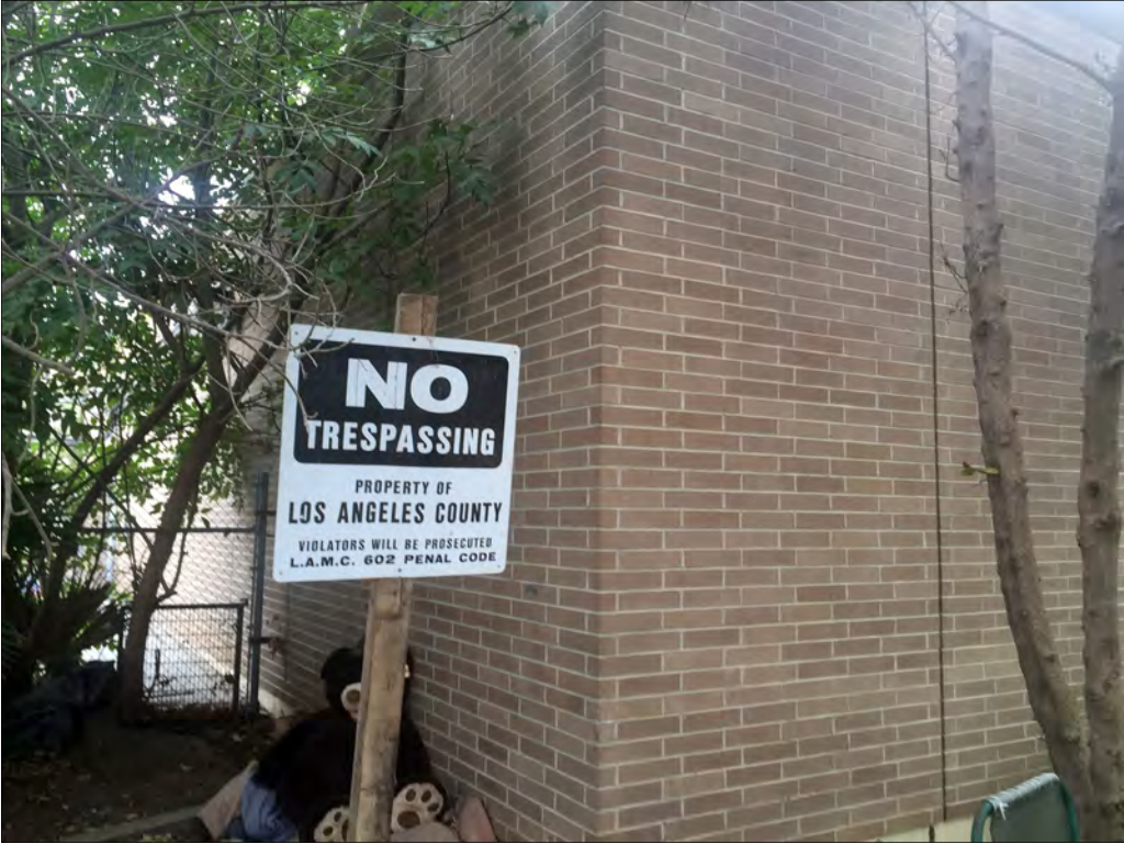
Figure 12: Sheriff's Station, west elevation (left) and south elevation (right), view northeast (Heumann, 2015)
