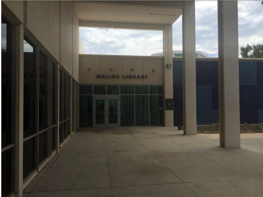
Figure 33: Library, west elevation, view east (Heumann, 2015)
