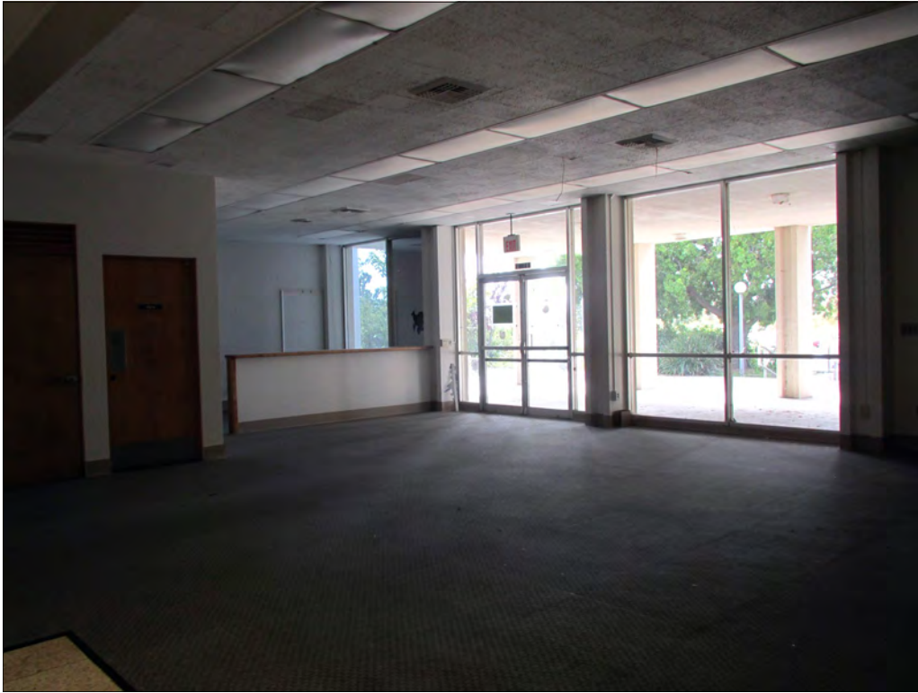
Figure 15: Sheriff's Station, main entry interior, view southwest (Heumann, 2015)
