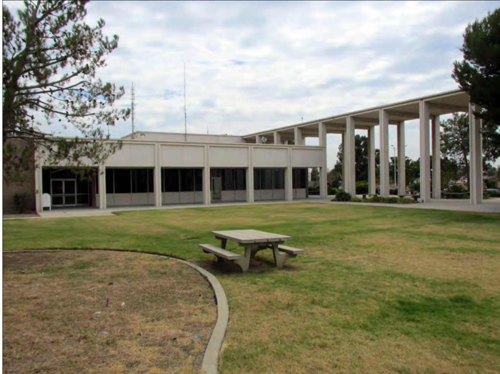
Figure 21: Water district, east elevation, view southwest across courtyard (Heumann, 2015)
