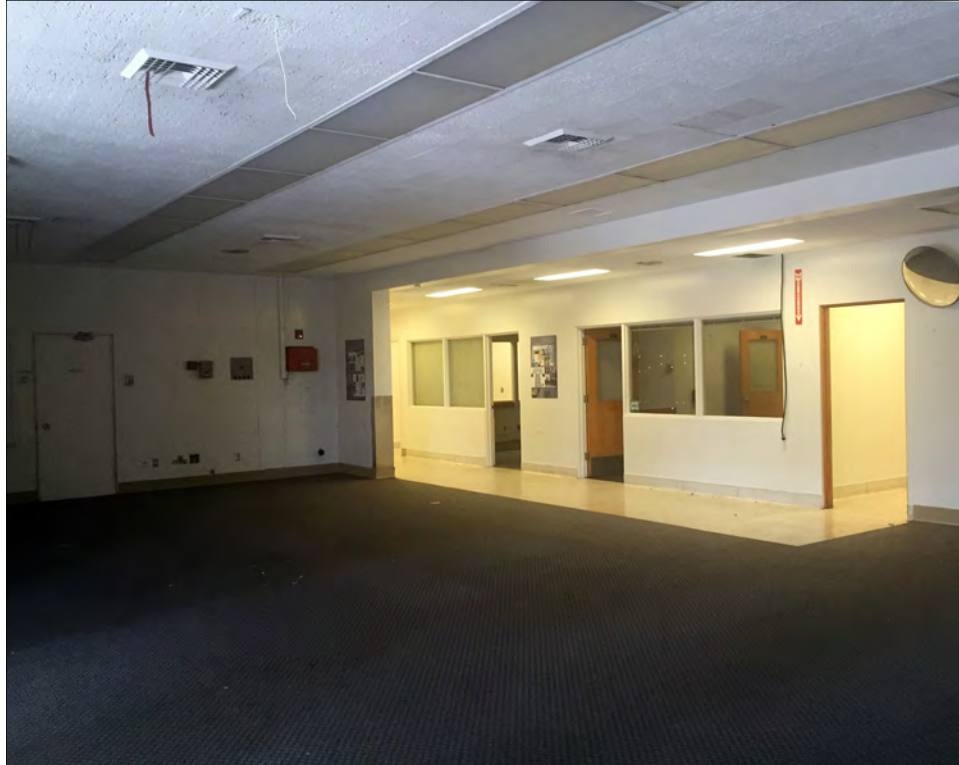
Figure 16: Sheriff's Station, main entry interior, view northwest (Heumann, 2015)
