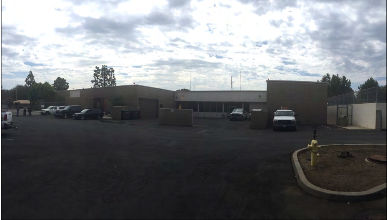
Figure 22: Water district (right) and Courthouse (left), north elevation, view southeast (Heumann, 2015)
