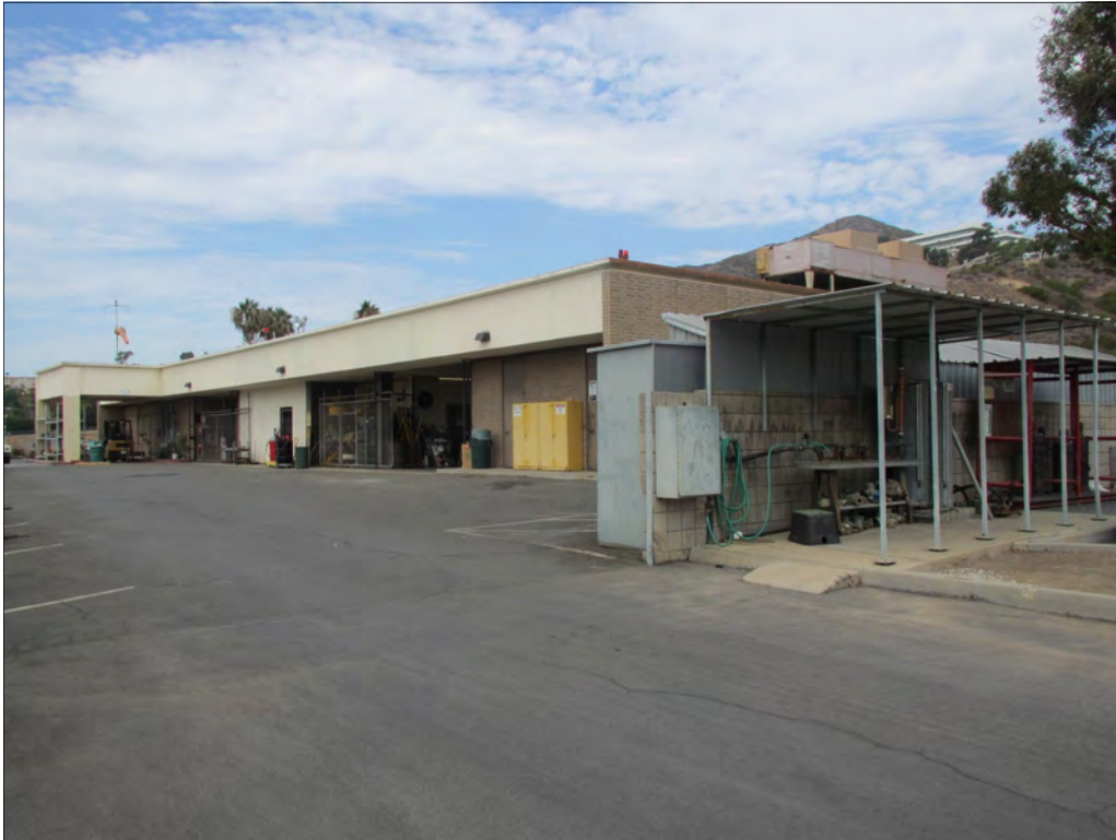
Figure 38: Maintenance, south elevation, view northwest (Heumann, 2015)
