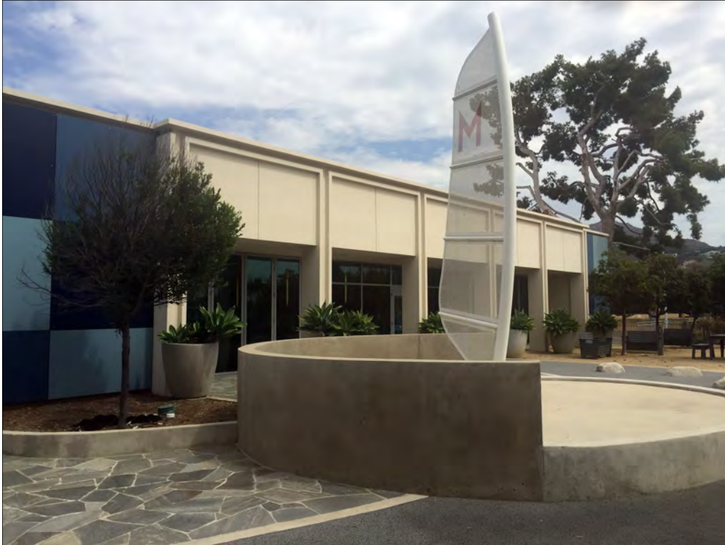
Figure 35: Library, south elevation, view northeast (Heumann, 2015)
