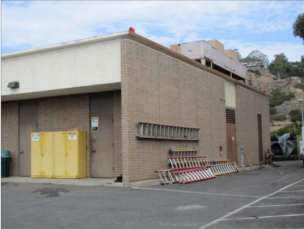
Figure 40: Maintenance, east elevation, view northwest (Heumann, 2015)
