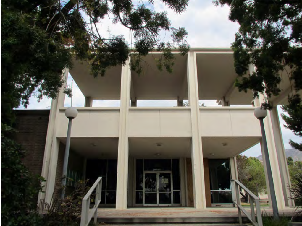
Figure 10: Sheriff's Station, south elevation, main entrance, note continuation of arcade, north view (Heumann, 2015)
