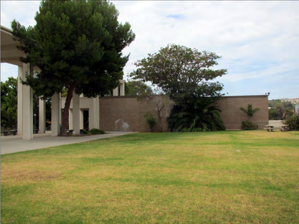
Figure 14: Sheriff's Station, east elevation, view west across courtyard (Heumann, 2015)
