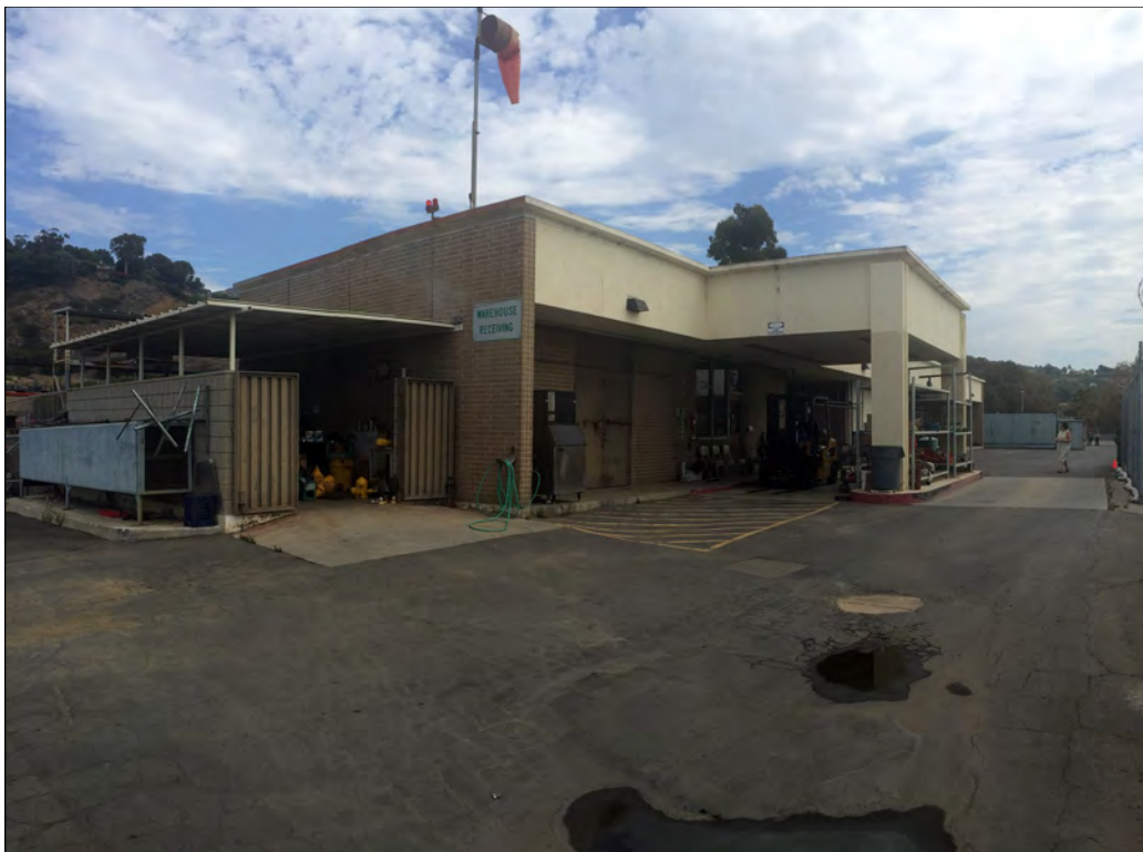
Figure 39: Maintenance, west elevation (left) and south elevation (right), view northeast (Heumann, 2015)
