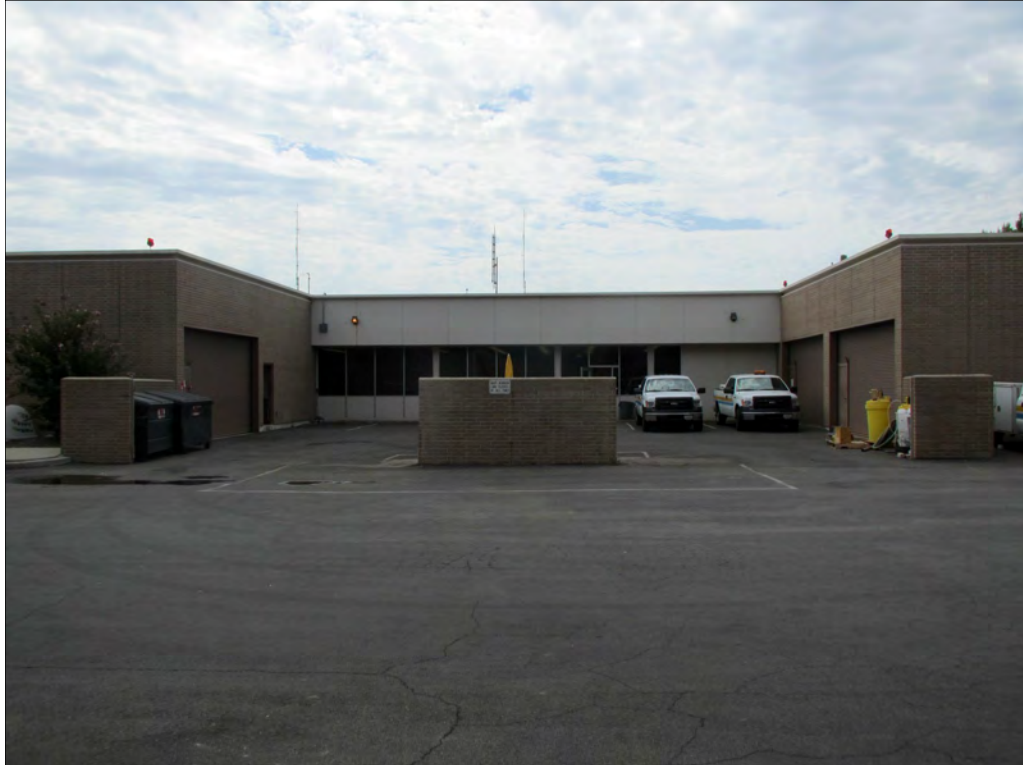
Figure 23: Water district, north elevation, view south (Heumann, 2015)
