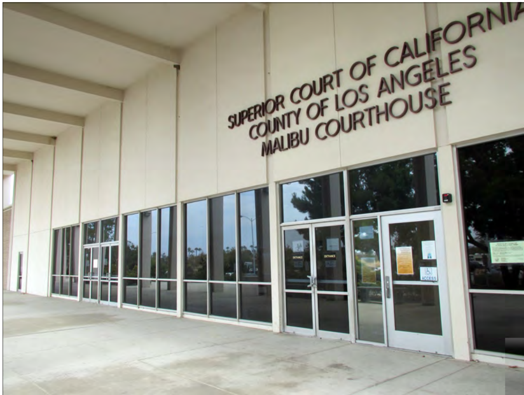
Figure 27: Courthouse, south elevation, view northwest (Heumann, 2015)
