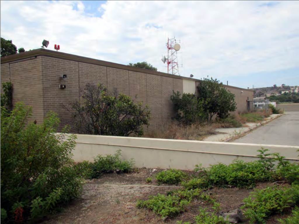
Figure 13: Sheriff's Station, north elevation, view southwest (Heumann, 2015)
