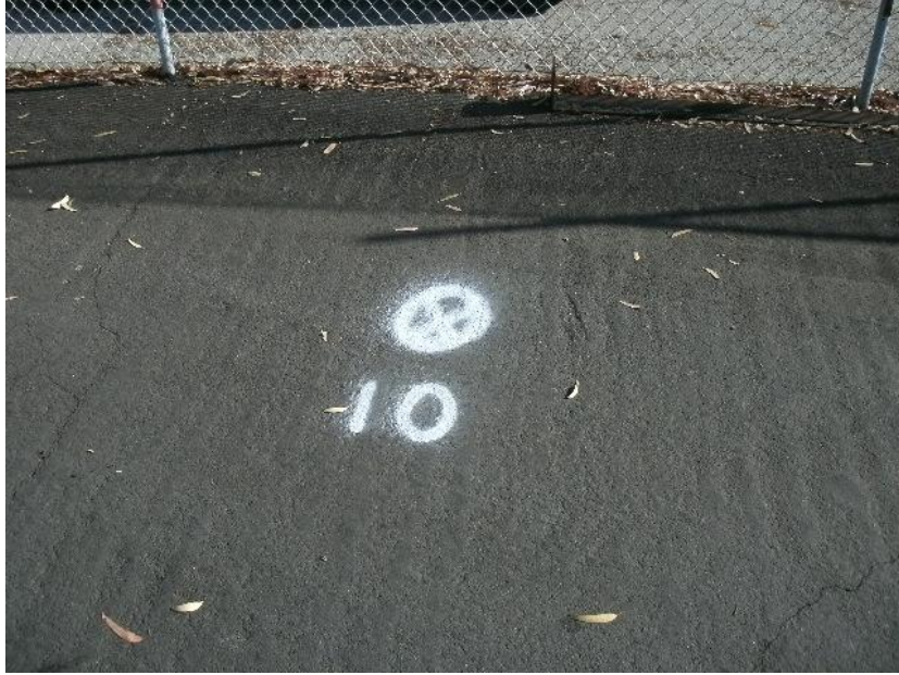
Photo 10: SB10 – Water Works parking lot.
