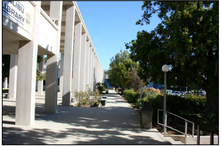
View 10: View of the Civic Center colonnade looking east from the Sheriff's Substation entrance.
