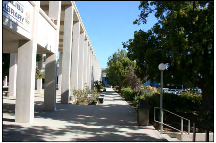
View 10: View of the Civic Center colonnade looking east from the Sheriff's Substation entrance.
