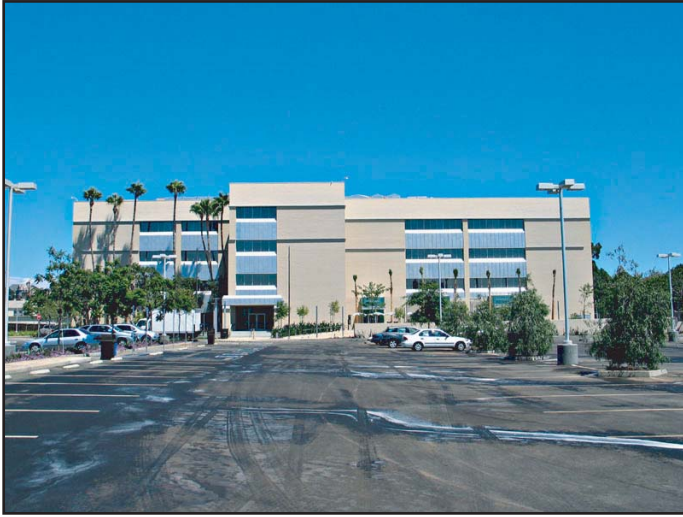
View 1: Looking east at the western face of the four-story West Building.
