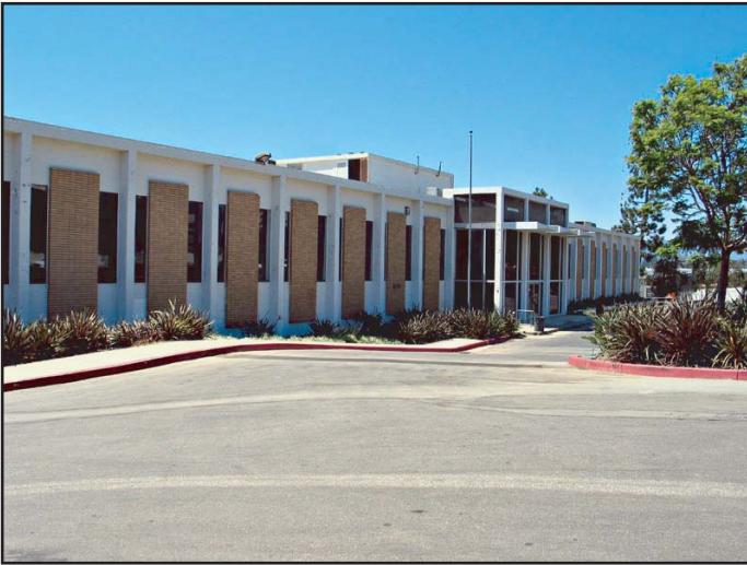
View 6: Looking north from the Bundy driveway at the east face of the vacant two-story building.
