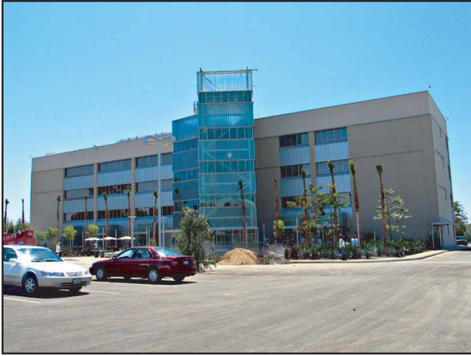
View 4: Looking west at the east face of the four-story building.
