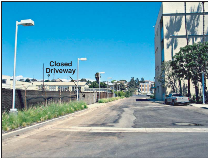
View 9: Looking east along the chain-link fence that forms the northern boundary of the Bundy Campus. To the left (north), a driveway is shown that once provided access to the site under BAE Systems ownership and is now closed.
