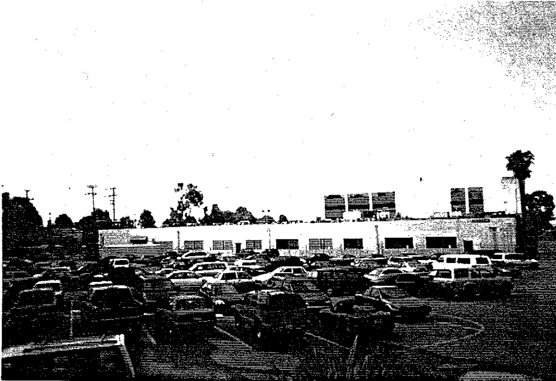
Photograph 1. Eastside of Building 1 and east parking Lot
