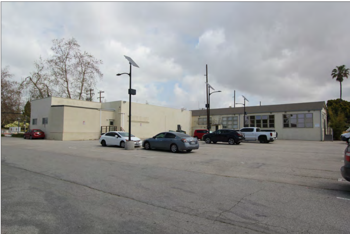
Image 8: Subject property, south elevation of main wing (left) and west elevation of gabled wing (right), view northeast (Chattel, 2023).
