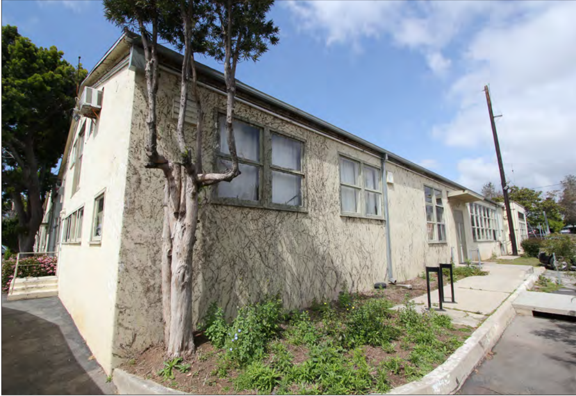
Image 15: Gabled wing, south (left) and east (right) elevations, view northwest (Chattel, 2023).
