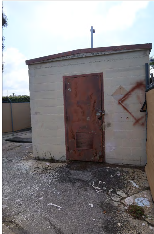
Image 25: Ancillary Building C, north elevation, view south (Chattel, 2023).
