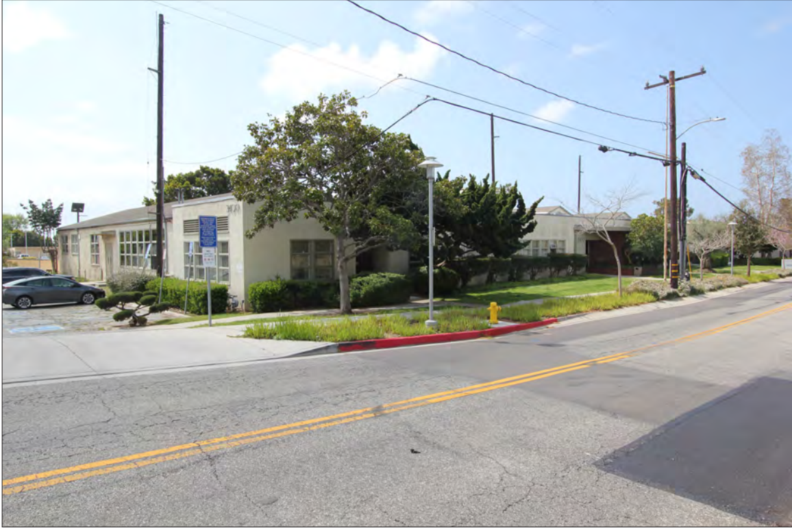
Image 1: Subject property, east (left) and north (right) elevations, view southwest (Chattel, 2023).
