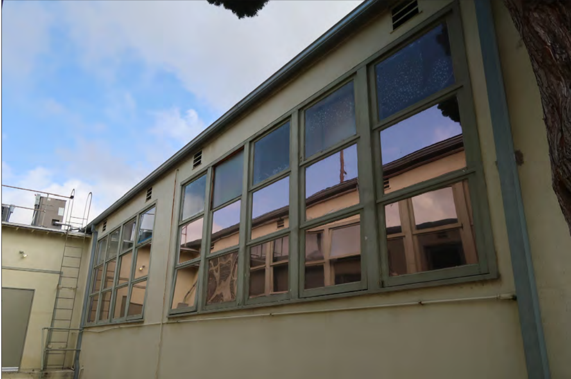
Image 19: Detail view of typical window at gabled wing, view northeast (Chattel, 2023).
