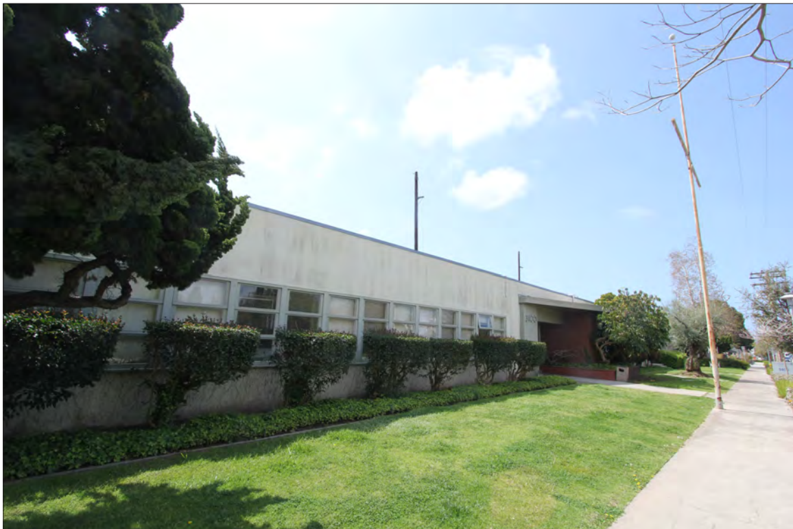
Image 2: Subject property, north elevation, view southwest (Chattel, 2023).
