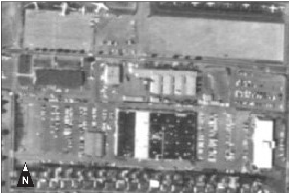
Image 12: Detail aerial view of subject property (UCSB Air Photo, 1962).
