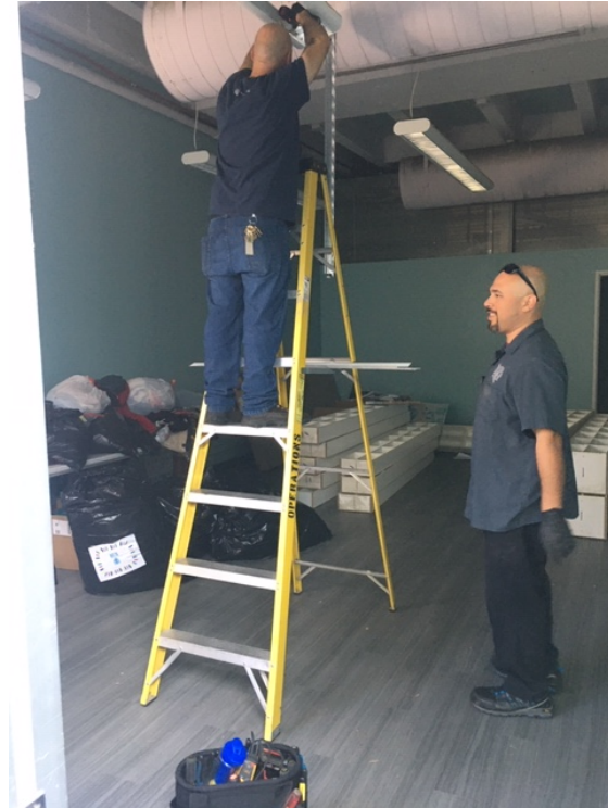
SMC New Food Pantry Under Construction
