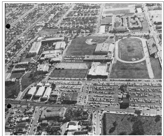
Figure 2 – Aerial photograph of main campus, circa 1962.
